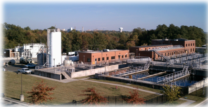
Jones Ferry Road Water Treatment Plant
