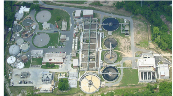
Mason Farm Wastewater Treatment Plant
