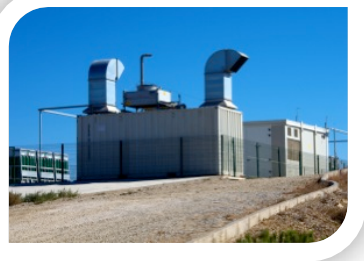
Bozcaada Island community powering
